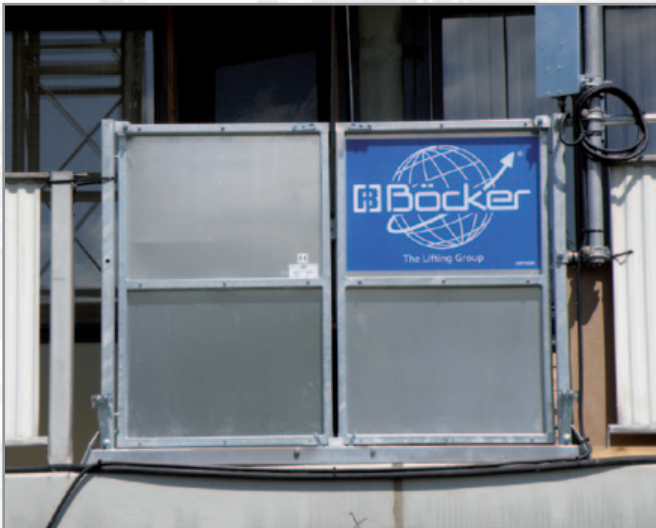
All landing gates comply with machinery directive 2006/42/EG
