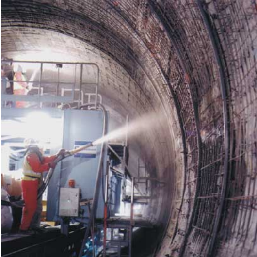
Two AL-246 spraying concrete by hand
